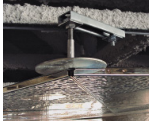
A specially developed fixing system gives great flexibility in fitting together the panels.
