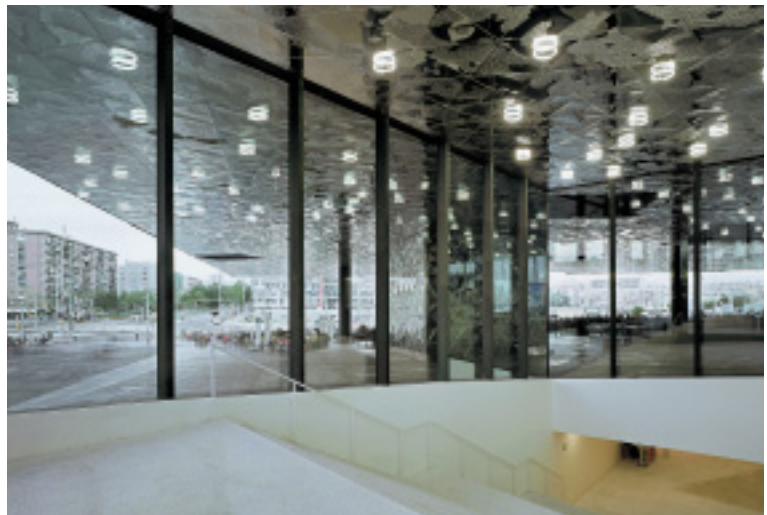
Broad expanses of glass and the use of stainless steel panelling on ceilings inside and out give an impression of continuous space.
