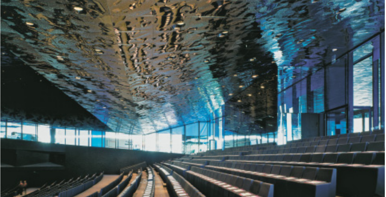
The stainless steel cladding seen outside continues in the auditorium on the underside of the balcony. The panels here have been coloured blue in an electrolytic process.
